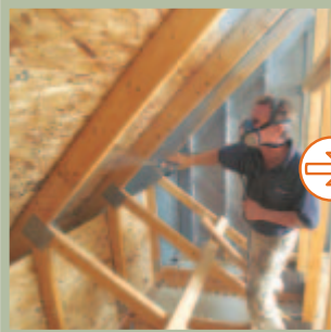
Spray and coat attic roof deck
