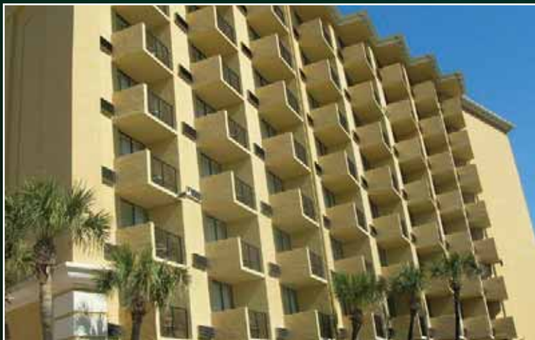
To ensure a long-lasting finish at the Nine Island Avenue high-rise condominium (above center and page 25), J.B. Painting chose a two-coat system of Loxon Masonry Primer and Coating. A final topcoat of SuperPaint Exterior Latex Satin provided the sheen the client wanted. Commercial projects include the Acapulco Hotel and Resort (above left) and the Plaza Resort and Spa (above right), both in Daytona Beach.
